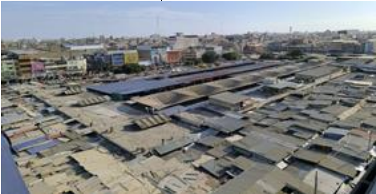
View of the roof of the Mercado Modelo in Chiclayo
